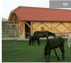
Hlevski objekt | The Stock Shed
