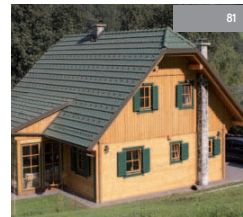
Stanovanjska hiša Pfeifer | The Pfeifer Residential House
