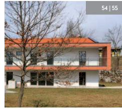
Pasivna hiša pri Divači | The Passive House near Divača
