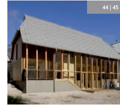
Popotresna obnova | Post-Earthquake Renovation
