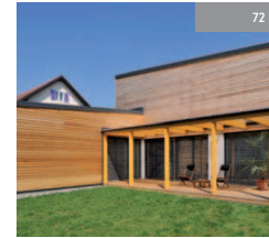
Pasivna hiša v Mariboru | The Passive House in Maribor
